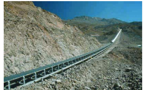
An uncovered section of the Overland Conveyor System at Minera Los Pelambres, Chile
